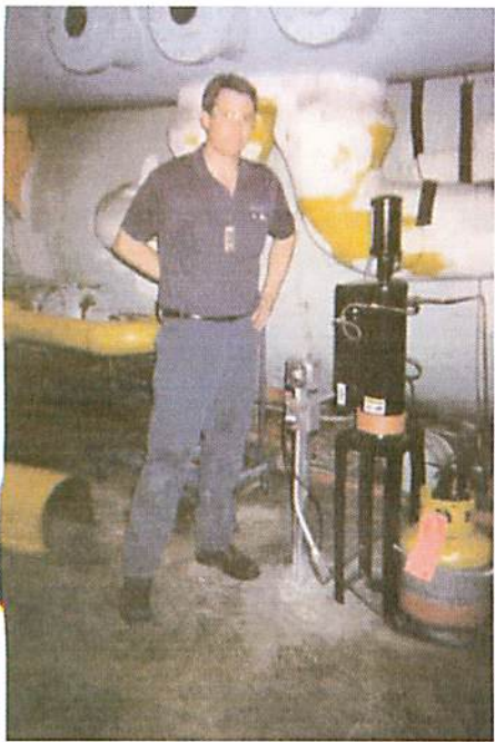
OAM-Purgers installed by Greg Beyer, Service Technician and David Holmquist, Technical Manager Central Chillers, from Owens Service Company, on a 5,500 ton chiller and on a 3,500 ton chiller at 3M facility Minnesota
